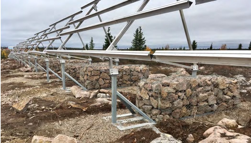
Figure 13: Solar arrays anchored with gabions – for uneven surfaces or when ground cannot be penetrated
