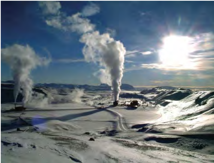
Figure 229: Krafla geothermal power plant in Iceland 256
