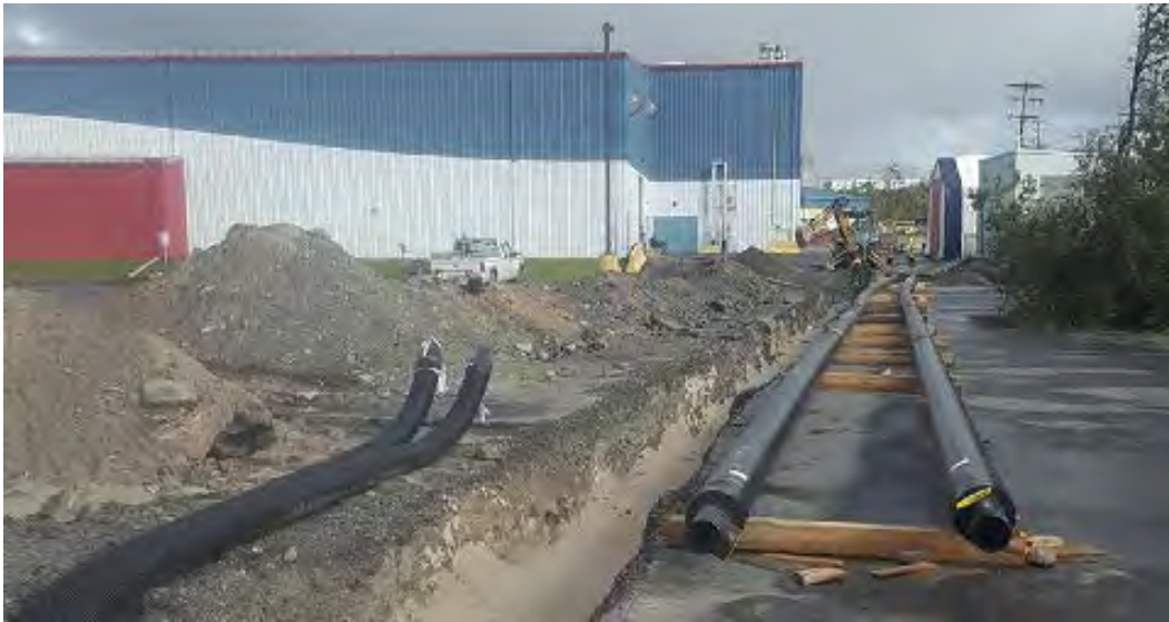
Figure 89: Installing district heating system in Yellowknife 111
