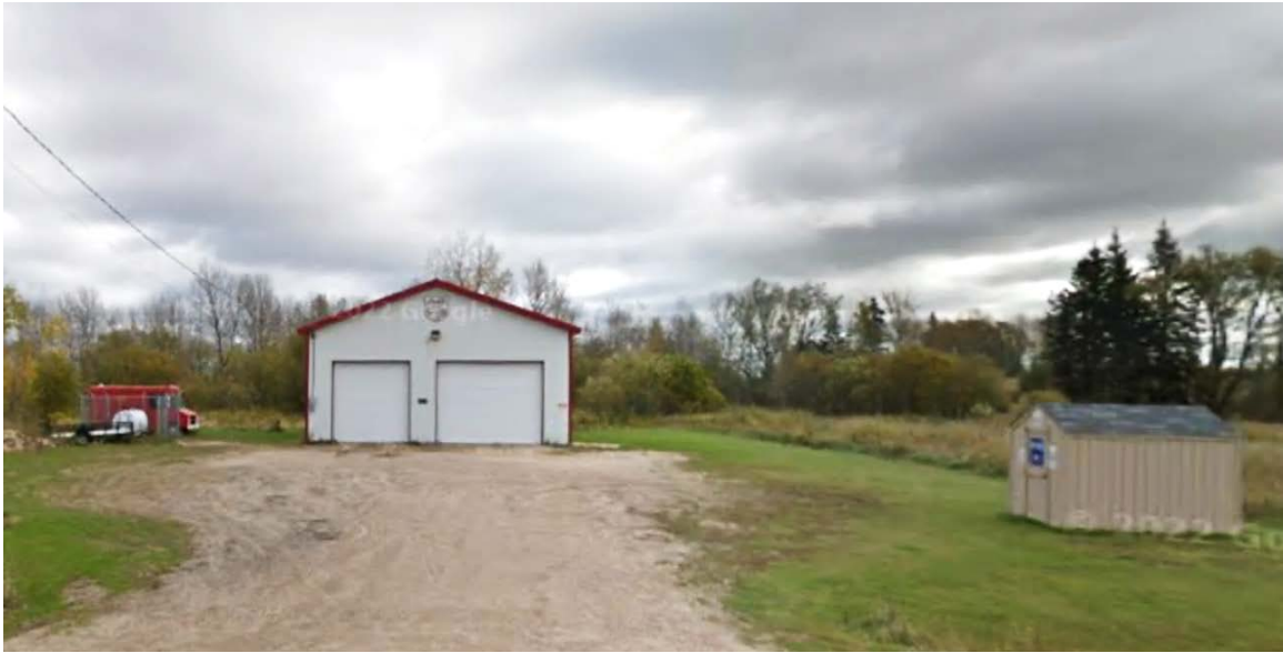
Figure 55: Fire Station 1, Piney, Manitoba – street view
