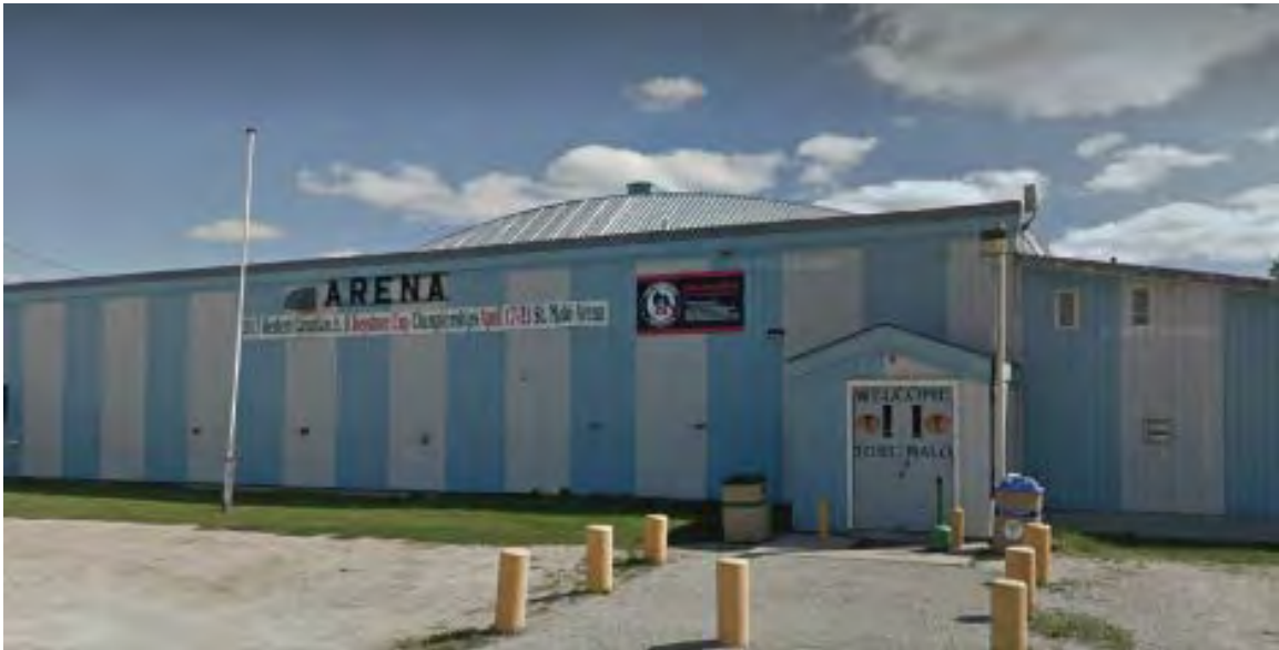
Figure 34: St. Malo Arena (De Salaberry Recreation Facility) – street view
