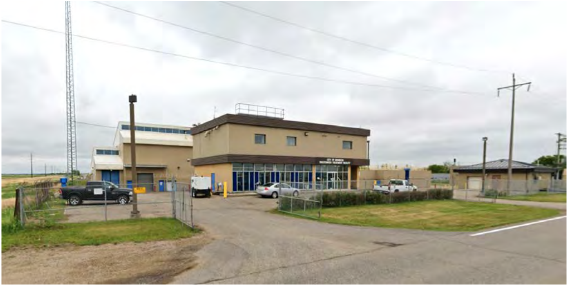
Figure 8: Brandon – Wastewater Treatment Facility – street view
