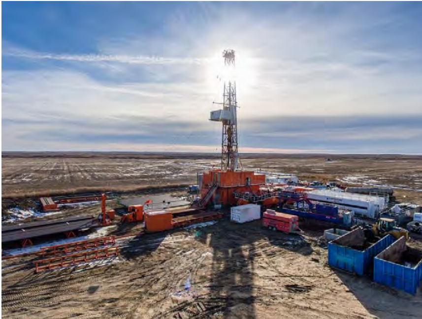
Figure 232: Drilling rig at the DEEP project site
