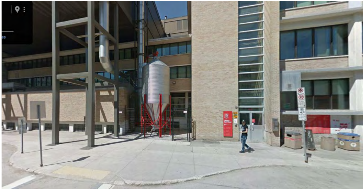
Figure 29: University of Winnipeg Biomass System Pellet Fuel Silo
