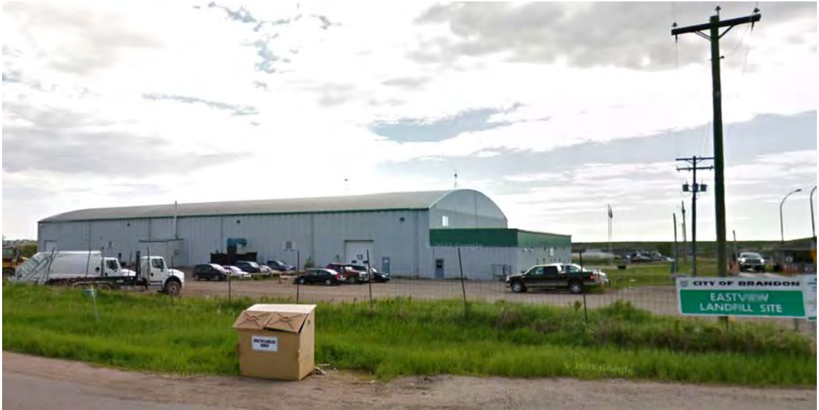
Figure 7: Brandon – Material Recovery Facility – street view
