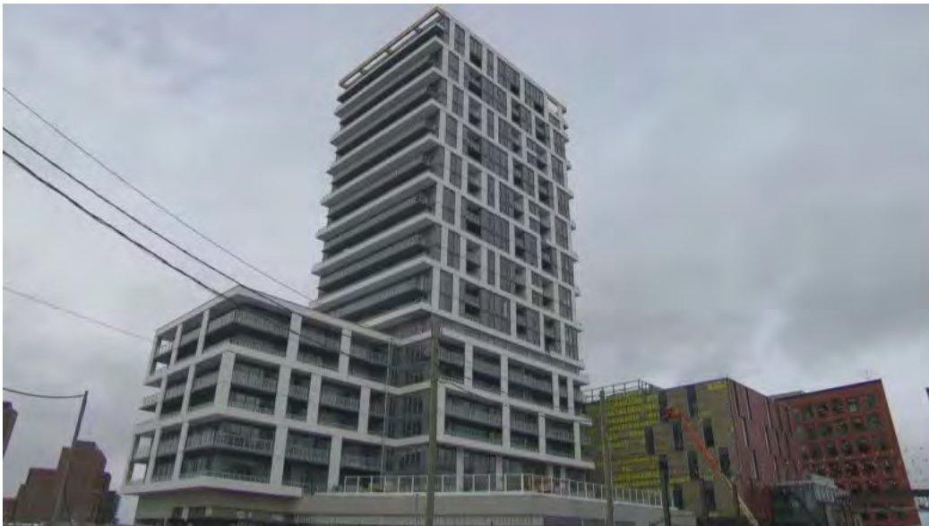
Figure 103: Common at Zibi – building heated with waste process heat
