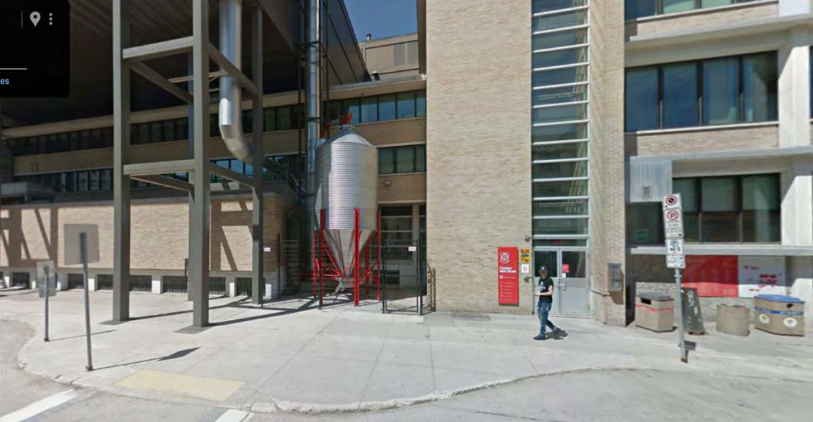
Figure 80: University of Winnipeg Biomass System Pellet Fuel Silo
