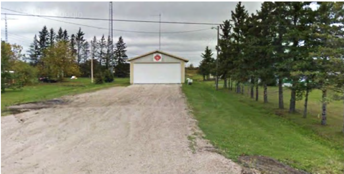
Figure 56: Fire Station 2, Sprague, Manitoba – street view
