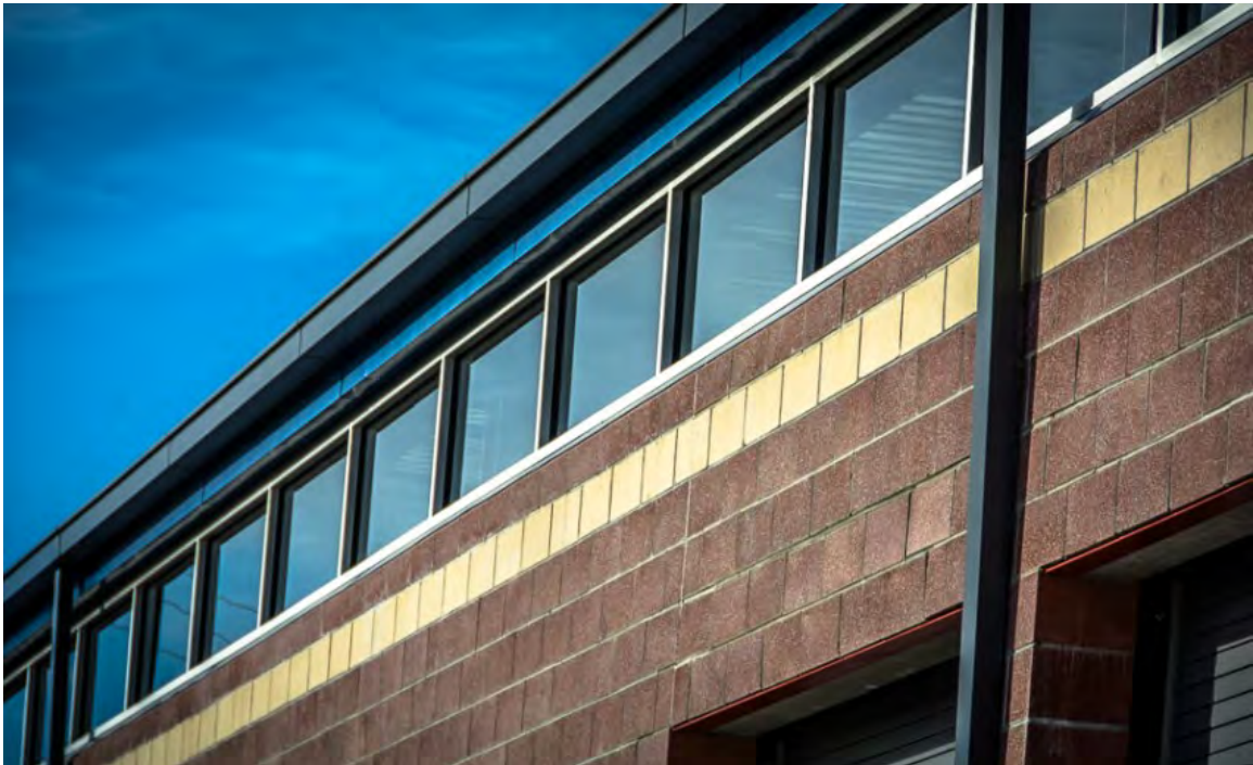
Figure 42: Clerestory windows on industrial building 45
